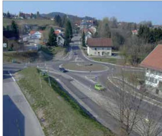
A roundabout unambiguously determines the right of way situation and reduces the speed level and thus the severity of accidents.
