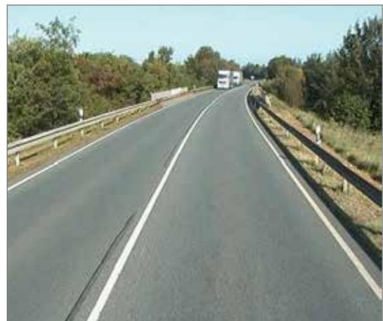
The solid line centre road marking prohibits overtaking and thus reduces the speed level.
