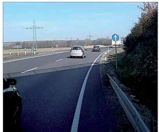
The new layout of the right road edge with a continuous radius and an increased consistent transverse slope eliminated the accident hotspot.
