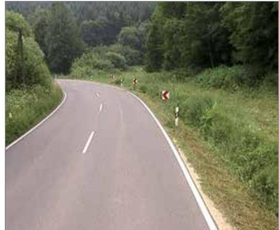
Additional individually placed bend chevrons make the direction of the bend clearer. **BUT:** Visibility is still limited by the vegetation in the inner bend.
