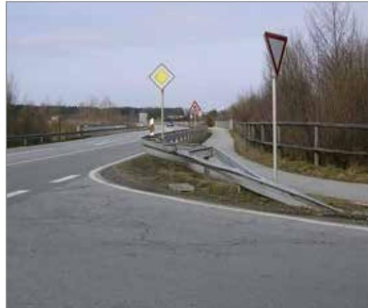
Visibility for traffic turning into the major road was improved by removing the vertical extension rail.
