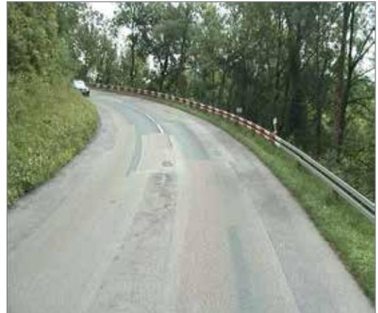
Traffic guidance equipment installed on top of the steel crash barrier makes it easier to see the direction of the bend.
