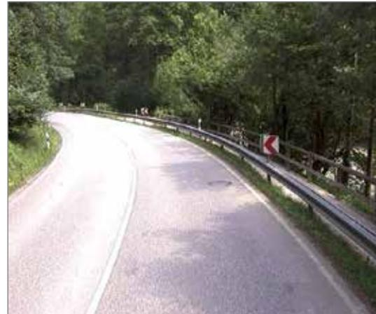
Individually placed bend chevrons indicate the direction of the bend. When a vehicle departs from the road, steel crash barriers prevent it from colliding with a tree which might have severe consequences.
