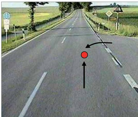
The stop line was no longer clearly visible causing vehicles to turn into the priority road without stopping and colliding with vehicles having the right of way.
