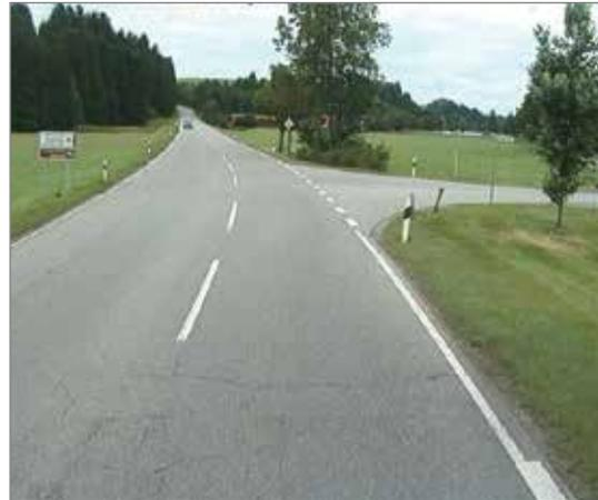
Obstructions reducing visibility for traffic turning into the major road were removed by optimising the installation sites of the signs.
