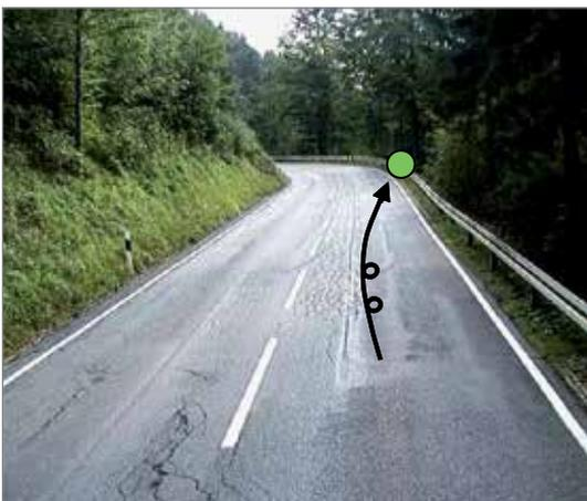
The road was in a very poor condition. In addition, it was very hard to identify the direction of the bend, which repeatedly resulted in single-vehicle accidents.
