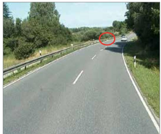
Thanks to the new wearing course, the road has more grip. In addition, the type II marking provides increased night-time visibility.
