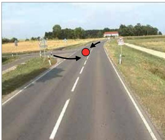
The intersection was hard to see in the dark. In addition, drivers drove too fast, which made it difficult for vehicles coming from the minor road to turn into the major road (short time gaps in the main flow).
