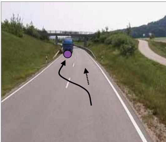
Visibility was insufficient for overtaking due to the slope and the bridge. However, drivers performed overtaking manoeuvres despite insufficient visibility, which caused severe accidents involving longitudinal traffic (rear-end and head-on collisions).
