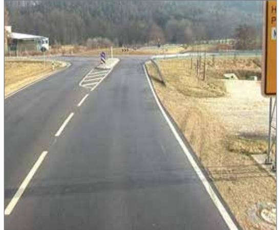
The conversion into a roundabout reduces the speed level at the intersection and makes turning into/crossing the major road easier (reduction of conflict points).
