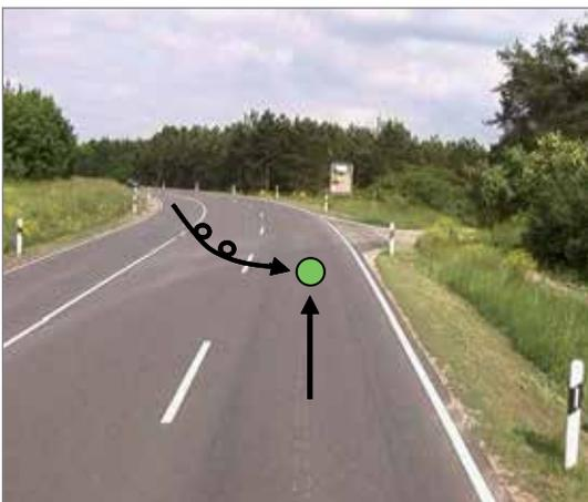
The single solid line centre road marking was insufficient to indicate the course and three-lane, single-carriageway layout of the road, which promoted single-vehicle accidents.
