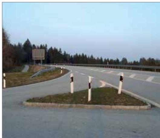
The steel crash barrier and the signs were set back from the edge of the road, which improves the visibility for traffic turning into the major road.
