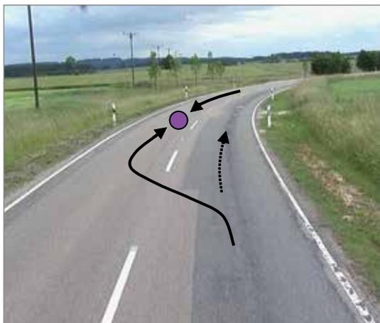
The course of the road was hard to see which is why the curvature of the road was underestimated. This repeatedly caused accidents involving longitudinal traffic (rear-end and head-on collisions) when overtaking.
